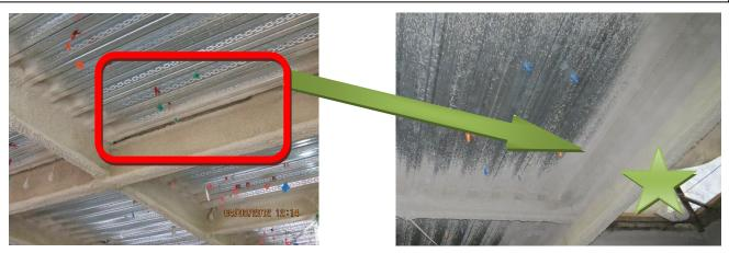
The flutes parallel to the top flange of the beam is required to be fully packed with spray fireproofing to the edge of the beam flange or other approved methods per NFCA Bulletin 1003.
