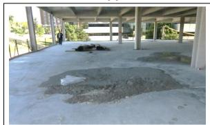
The floor should be covered with plastic in order to protect the floor from extra moisture from the spray fireproofing, which could create concerns with the floor finish.
