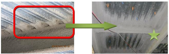
The flutes perpendiular to the top flange of the beam is required to be fully packed with spray fireproofing to the edge of the beam flange or other approved methods per NFCA Bulletin 1003.
